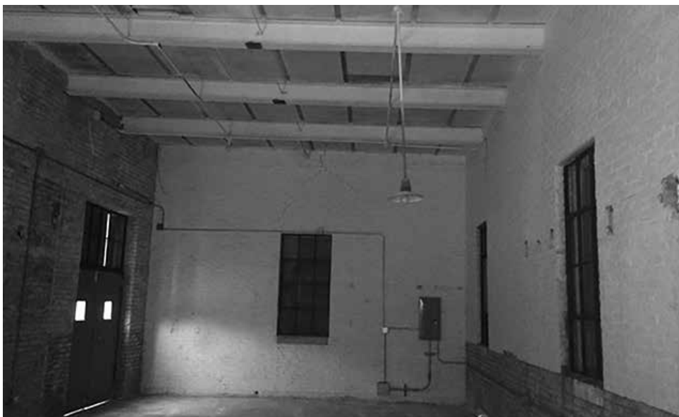
The interior of the Sparky Park building now that the steel beams (which used to hold electrical equipment) have been removed.
