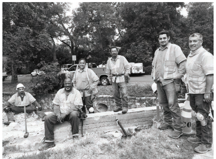
Photo of the Month: Hardworking Co.A Team Installs Sidewalks
