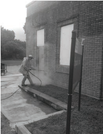
Cleaning the Building Before Construction
