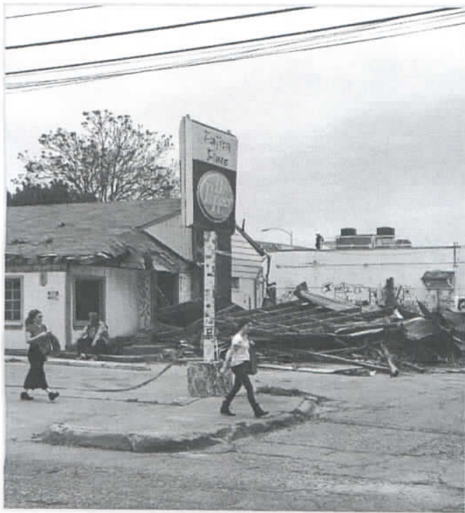
The demolished back portion of the former Ruby's BBQ
