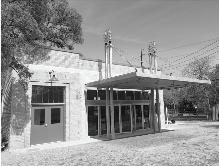
The Sparky Park building renovation is finally complete!
