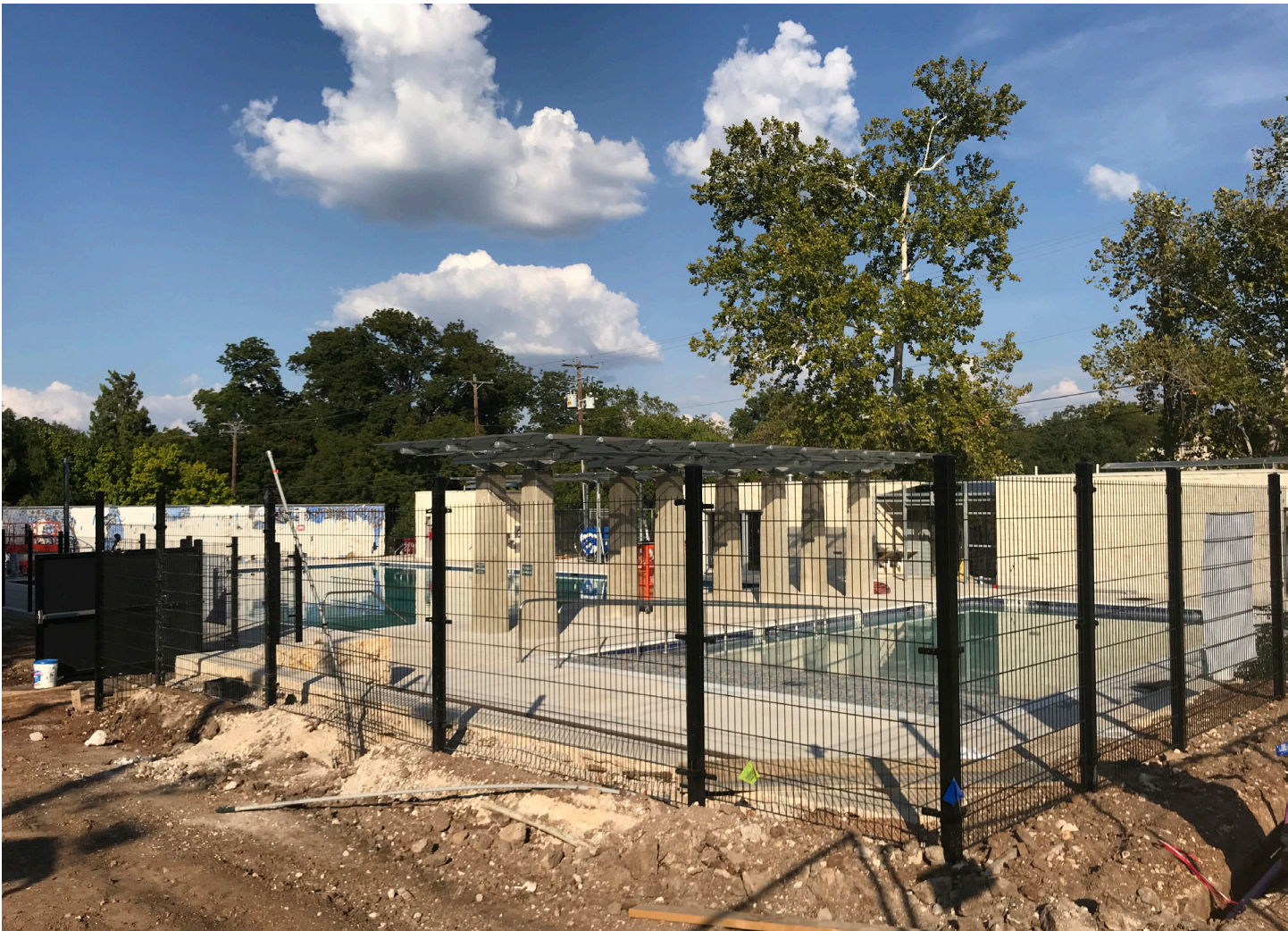
Shipe pool construction progress
